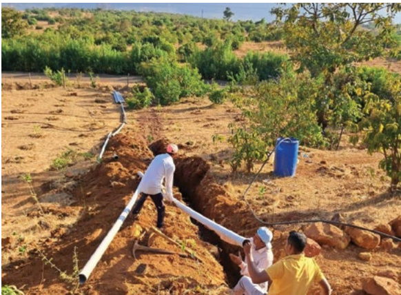
Pipeline Laying for Water Arrangements
